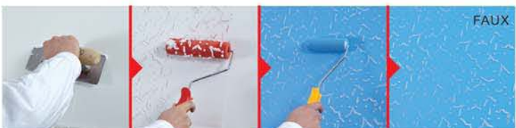
Step 1: Apply texture paint. Step 2: Before the texture paint is dry, roll the design roller from top to down. Step 3: After the texture paint is dry, paint the color.
