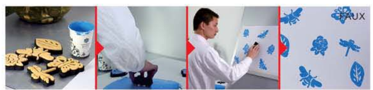
Step 1 : Prepare for the paint and rubber stamp. Step 2 : Absorb the color. Step 3 : Stamp on the surface create designs. Surface : The surface can be walls, furniture, fabric and paper.
