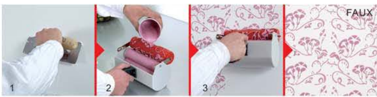
Step 1: Apply first color. Step 2: Put the paint into decoration machine. Step 3: Rolling form top to bottom, keep straight.
