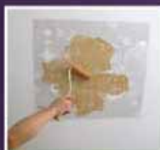
5. roll the paint on the stencil including the location hole.
